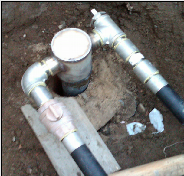
A stainless steel Rygan well head specially configured for data collection and monitoring.
