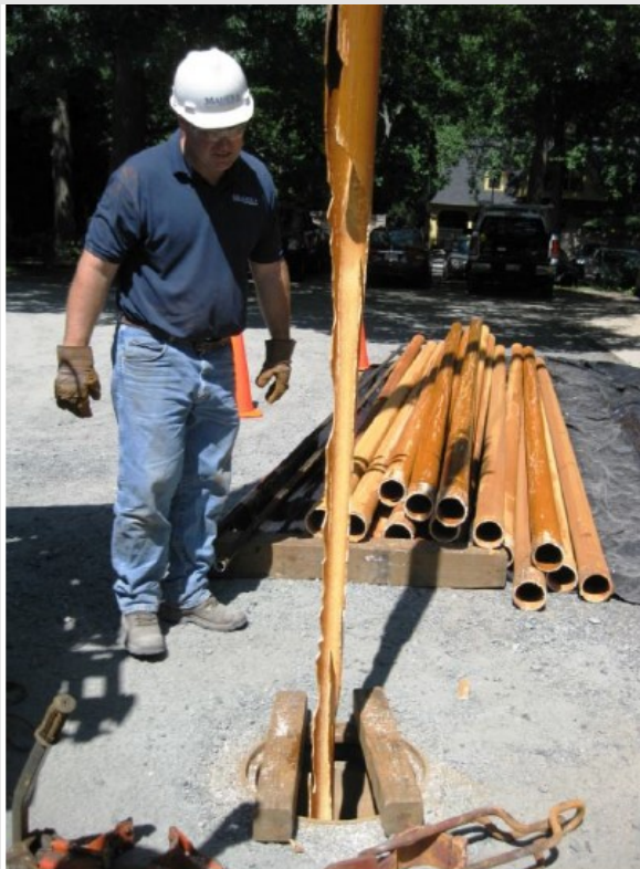
Collapsed porter shrouds of the failed system being removed, note the orange stain from iron fouling
