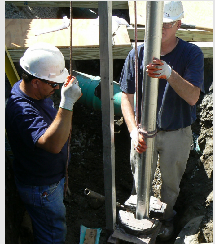
HPGX casing being lowered into a well bore
