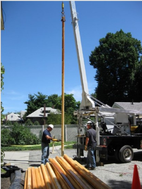
Collapsed porter shrouds of the failed system being removed, note the orange stain from iron fouling
